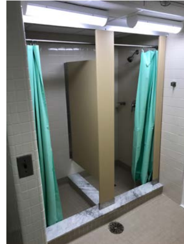
Typical Shower Area
