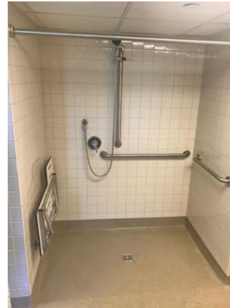
Typical Shower Area
