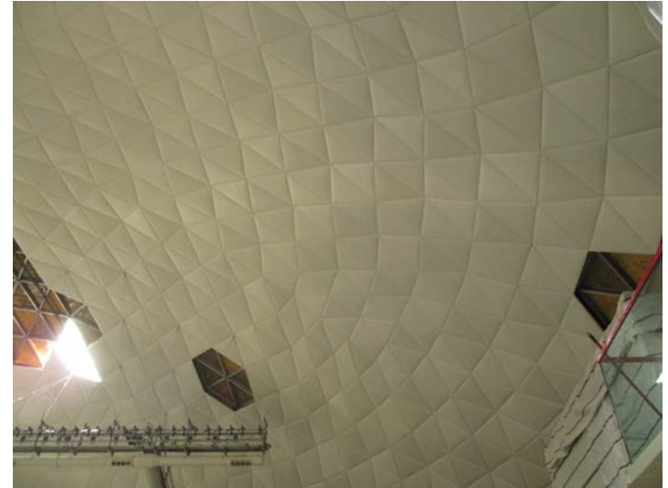
Progress of New Panel Replacement and Installation
