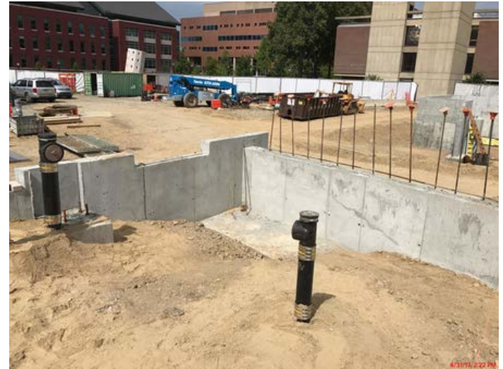
Foundation Wall with Utility Stub-Up
