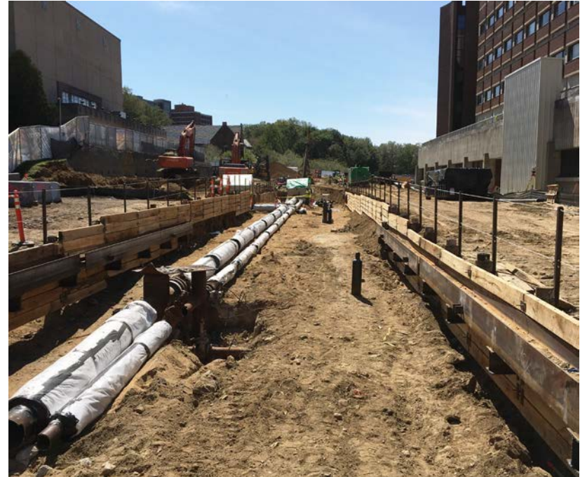
Utility Tunnel Excavation in Progress Jorgensen Auditorium on left, Gant Science Building on Right
