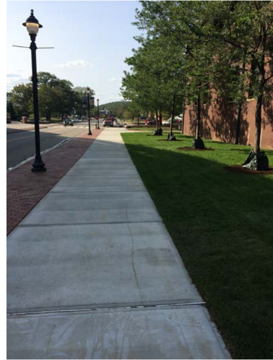
Site Restoration Complete
