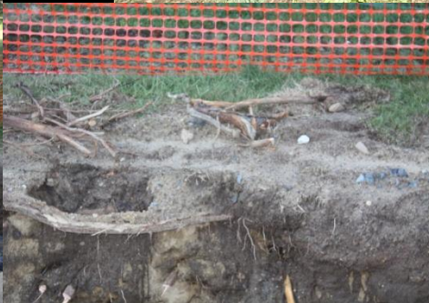
Excavation where roots severed on mature Cypress specimen
