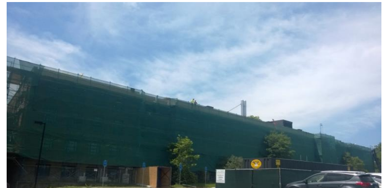
West façade of Young Building, top East façade of Young Building, bottom
