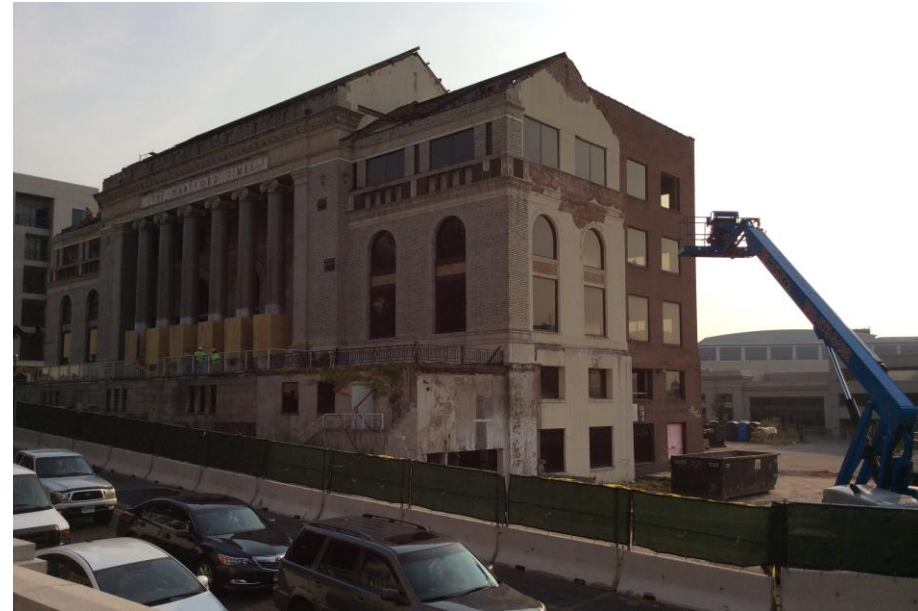
Construction on the Hartford Times Building
