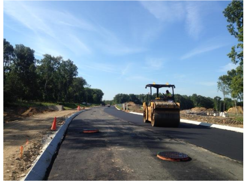
Final Paving in Progress
